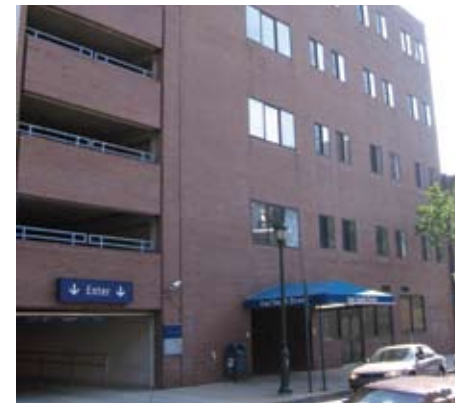
1740 South Street. The building's entrance, lobby and other public spaces were redesigned. Building mechanicals and all finishes were upgraded.
